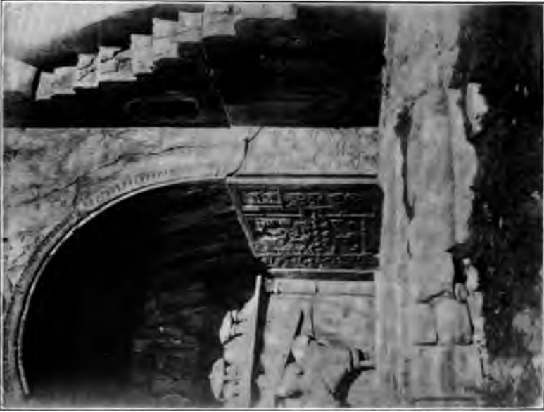
VIEW OF THE LARGER ARCH
